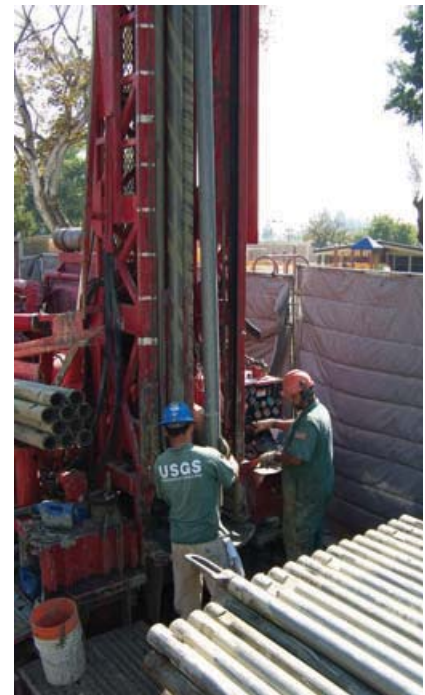
Figure 5. A team advances drill bit as one of the wells in the monitoring system is drilled.
